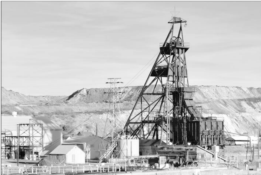
Bisbee, Campbell Shaft - headframe, ore processing buildings and tailings hill
